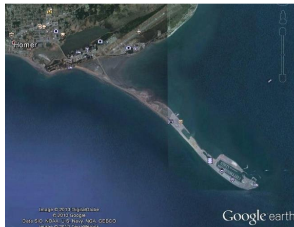
Figure 2. Aerial view of Homer Spit
